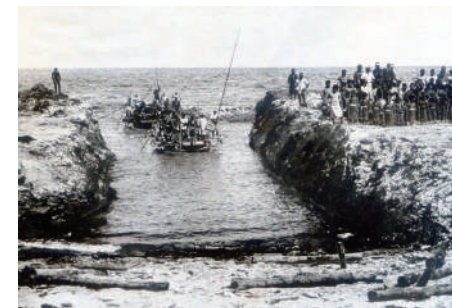
The landing on Uotsuri, created by blasting a rocky beach with dynamite.
